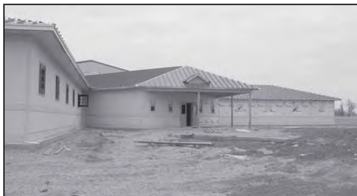
The exterior of the new facility is nearing completion.
